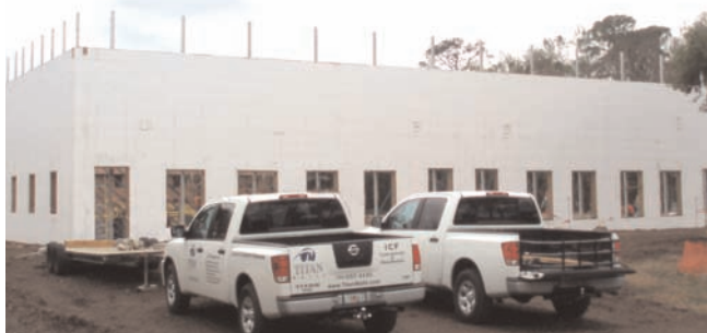
Above – 20ft high Amvic walls with 43 openings.
